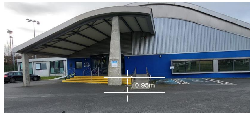
Fig. 3. Existing Front Entrance – Ground level to Finished Floor Level
